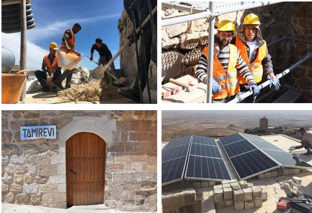
Figures 5.48- 5.51: Tamirevi and its construction process (KMKD, 2020).
