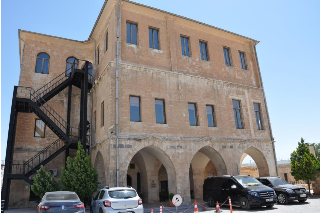
Figure 5.88: Mardin Artuklu University, Faculty of Architecture and Engineering, June 2021.
